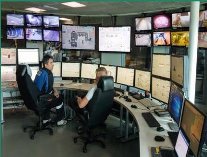
The control room of eco power plant, where staff monitor and control by huge claws the 2 large waste feeder bays that receives municipal waste 24 hours a day.
